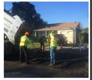
completedall work on the 2015 Street Resurfacing Repair Project on Friday, November 13,2015. The work included approximately 3,050 square feet of needed4-inch asphalt concrete roadway repairs on nine residential streets within the City of Pleasant Hill in anticipation of the winter rains.
