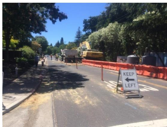
A one-way traffic control has been established for the westbound traffic along Westover Drive at the work zone, while eastbound vehicles along Westover Drive are being detoured along Lockwood Lane and Maureen Lane to avoid the construction work zone. A flagger will assist trail users through the construction area.
